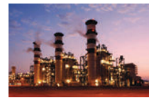
Mirfa Independent Water and Power Project Abu Dhabi, U.A.E.
